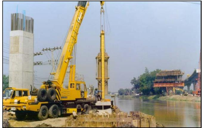
Figure 5. Dynamic load test carried out on a barrette (1.0m x 2.7m x 48.94m).
