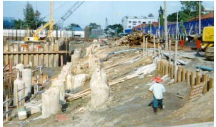
Figure 3. A picture showing slope excavation with sheet pile support – Case I
