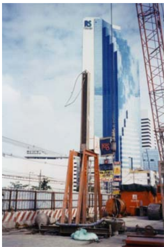
Figure 6. Guide frame for steel stanchion installation in barrettes
