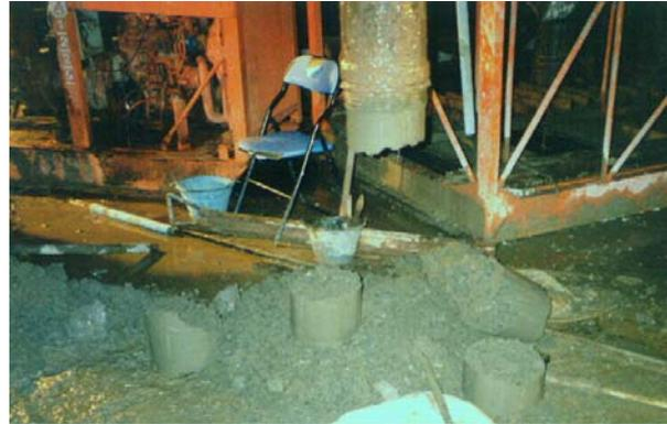
Figure 8. Tremie blocked by stiffening concrete
