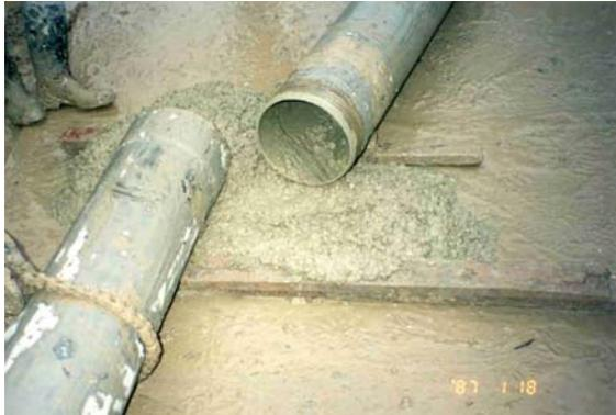
Figure 7. Tremie blocked by segregated concrete.
