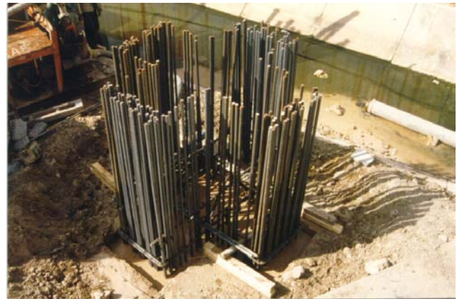
Figure 9. Reinforcement being installed in the trench
