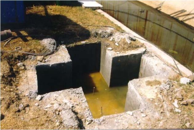
Figure 8. Guide wall for a cruciform barrette
