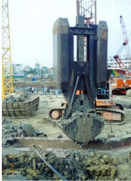
Diaphragm wall panel excavation.
