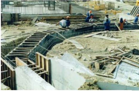
Guide wall construction.
