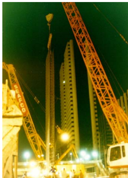
Installing a 20m-long reinforcement cage for a diaphragm wall panel.
