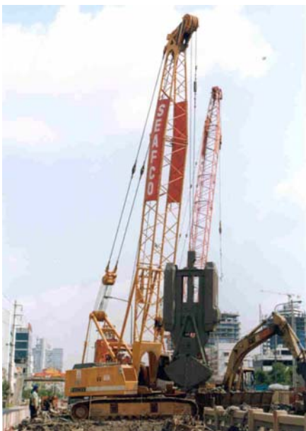
Diaphragm wall panel excavation.
