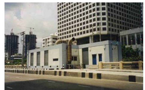
Sathorn pump station.
