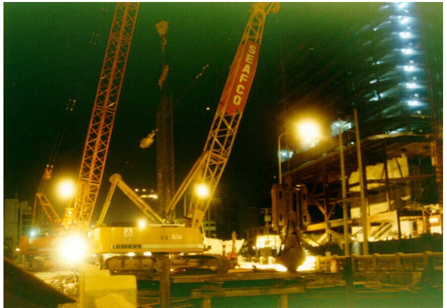
Diaphragm wall construction for Sathorn Pump Station.
