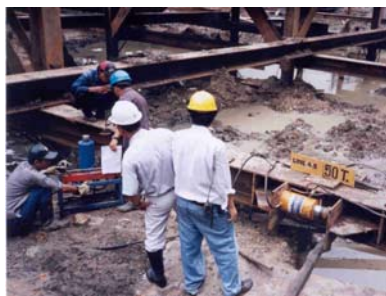
Pre-loading the struts.
