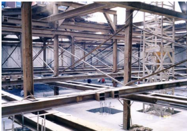
Excavation completed to the final depth.
