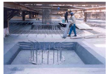
Preparation for base slab casting.
