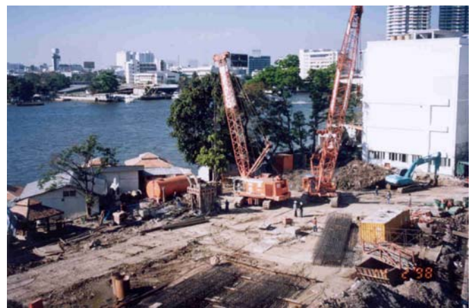
Diaphragm wall panel excavation.
