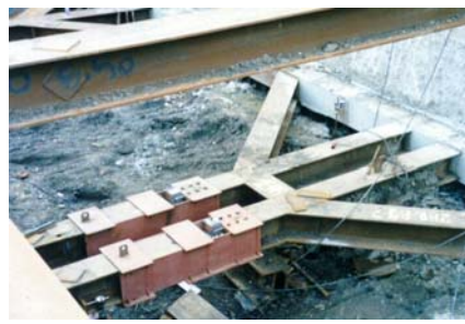
Earth pressure gauges for checking the strut force.
