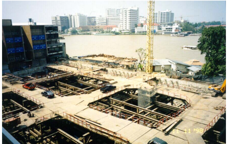
Temporary bracing and working platform.
