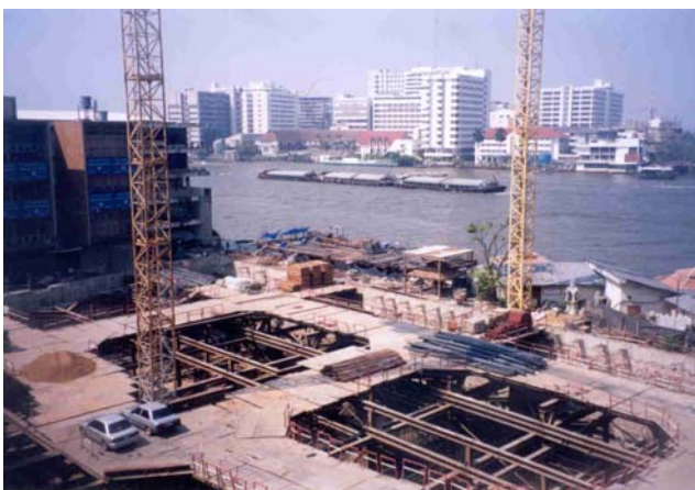
Excavation and basement construction.
