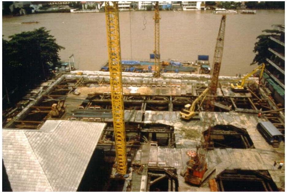
Temporary bracing for excavation and basement construction.
