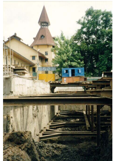
Excavation work in progress.
