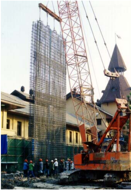
D-Wall work in progress.
