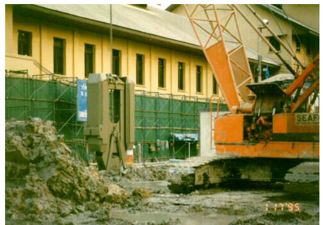
Diaphragm wall panel excavation.
