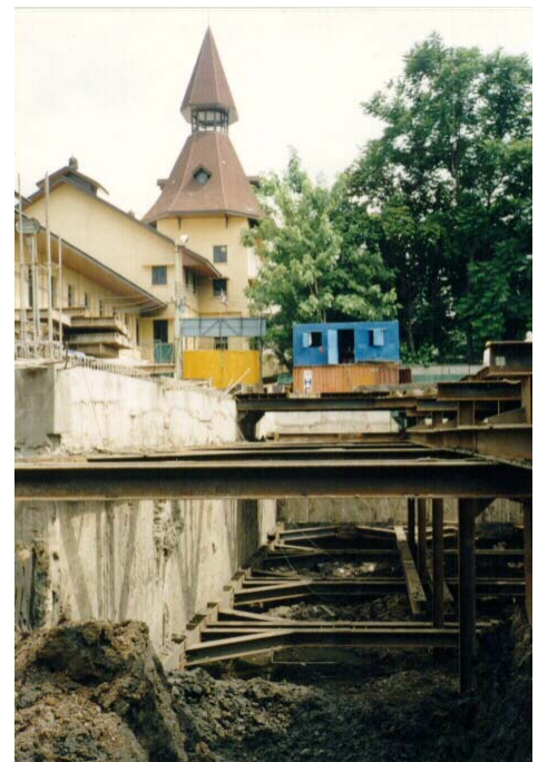
Excavation work in progress.
