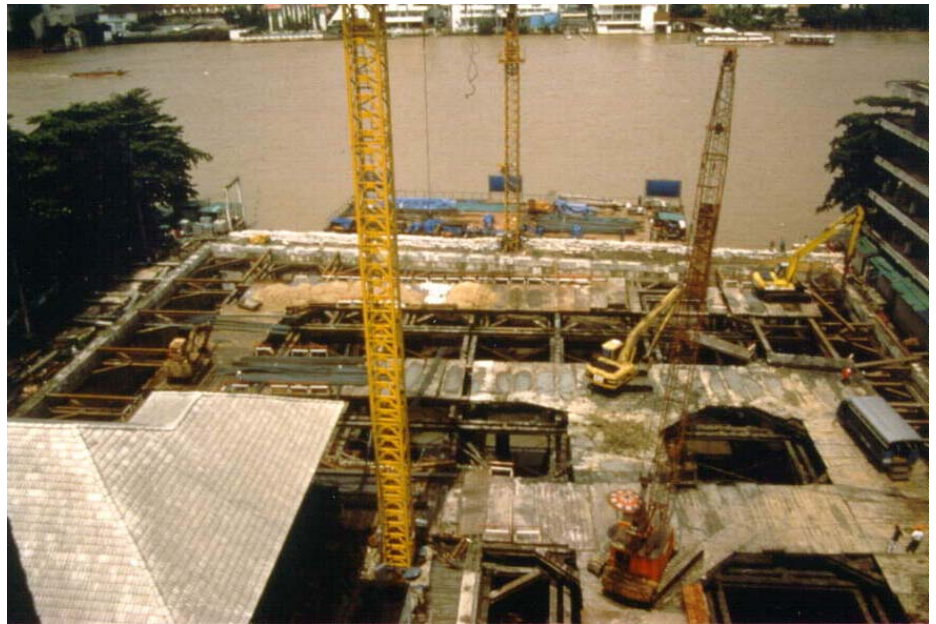
Temporary bracing for excavation and basement construction.
