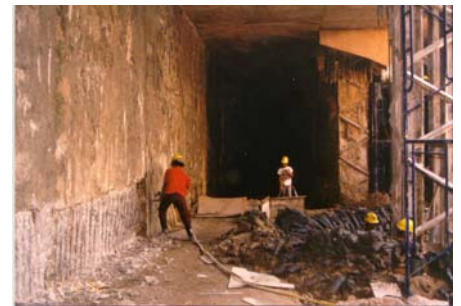
Preparation for connections between basement floor and diaphragm wall.
