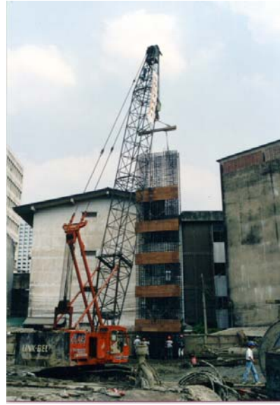
Lowering a rebar cage section with box-outs for basement slab connections.
