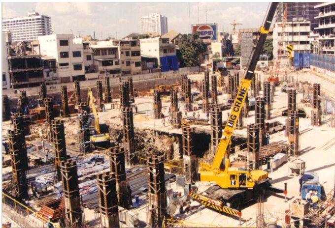
View of basement construction with top-down method.
