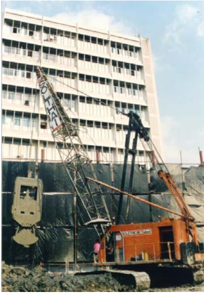
Diaphragm wall panel excavation.
