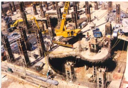
Excavation below the basement slab.
