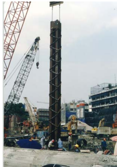
Installing a 24.0m-long built-up steel stanchion in the borehole.
