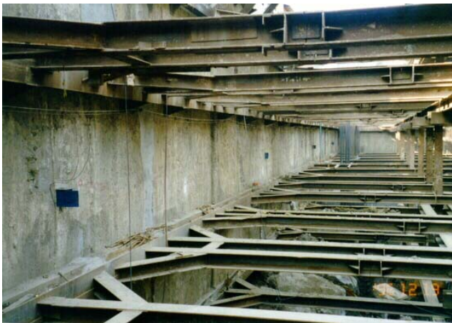
Exposed diaphragm wall.
