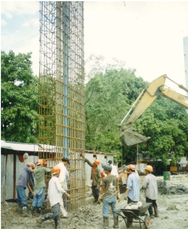
Lowering a reinforcement cage attached with inclinometer tube void former.
