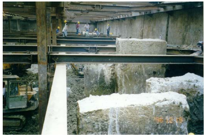
Exposed barrette top sections.
