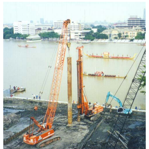
Piling in the main bridge area.
