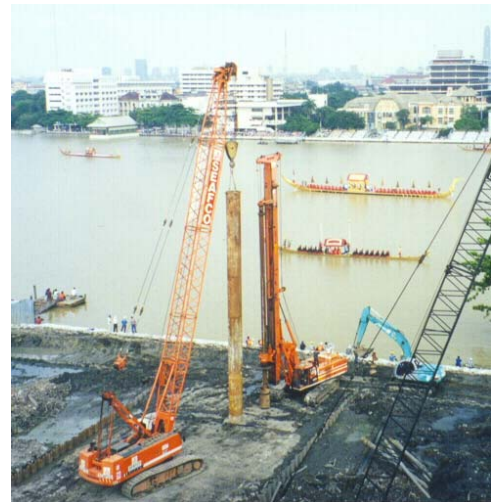
Piling in the main bridge area.
