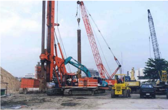
Bored piling in progress in the main bridge area.
