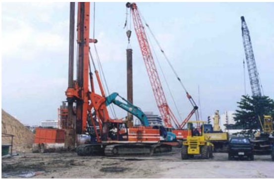
Bored piling in progress in the main bridge area.
