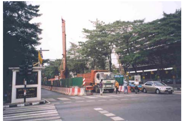
Piling in progress for the viaduct in front of the Bank of Thailand.
