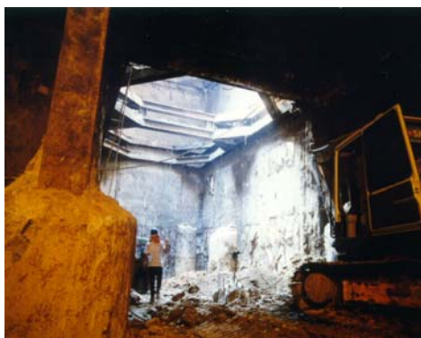
Excavation below the basement slab.
