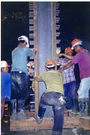
Lowering a steel stanchion into borehole before casting the pile.
