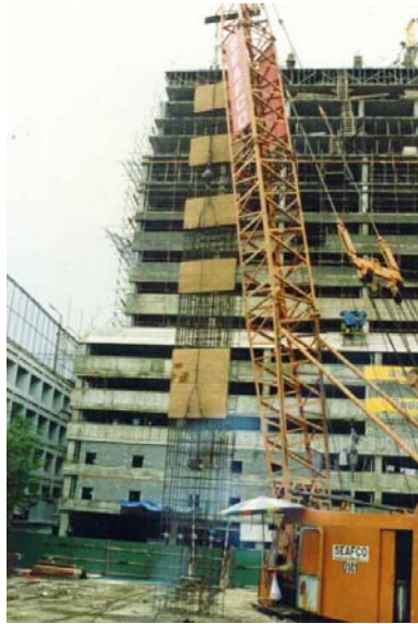
21m-long reinforcement cage with box-outs for basement slab connections.
