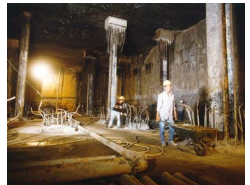
Excavation at final depth of 14.5m below ground level.
