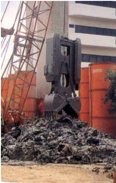
Diaphragm wall panel excavation.
