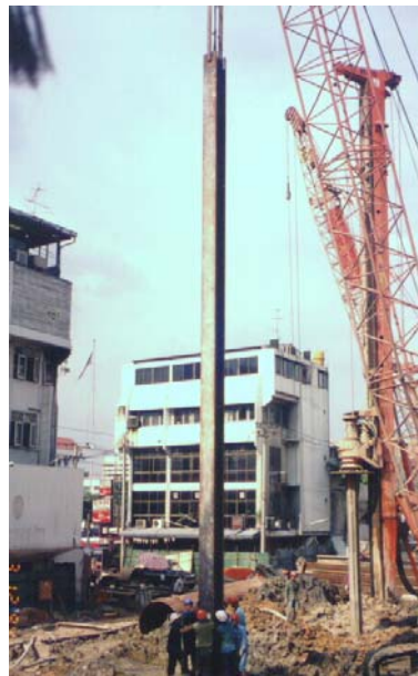
Installing a 18.0m-long steel stanchion in the borehole.
