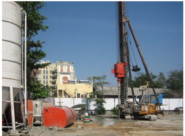
Deep soil mixing (soil-cement column works) in progress.
