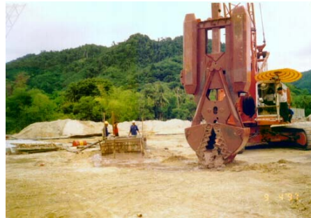
Excavation for a barrette.
