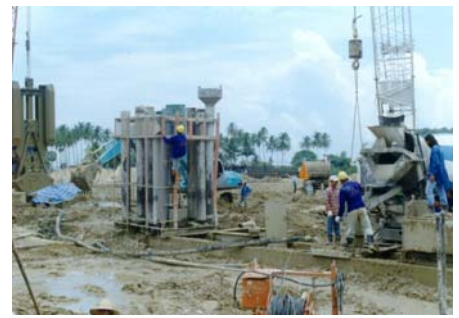
Casting a diaphragm wall panel.
