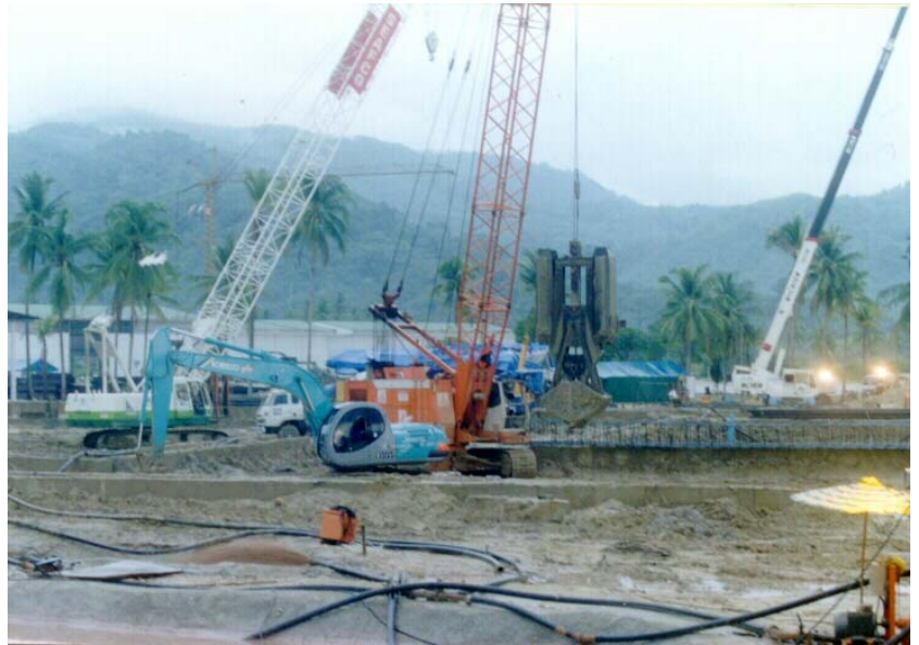
General view of diaphragm wall construction.
