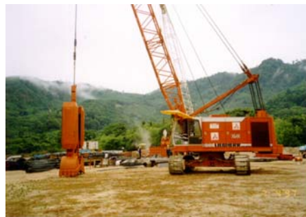
Clamshell grab for diaphragm wall and barrette work.
