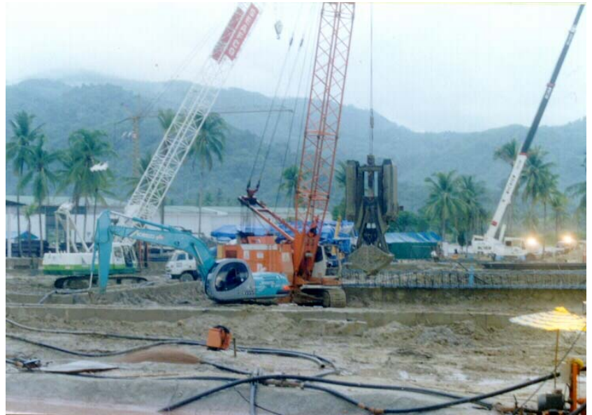
General view of diaphragm wall construction.
