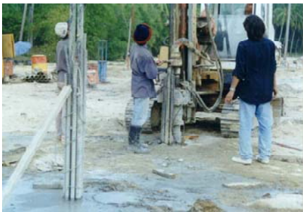
Anchor piles installation in progress (by other).
