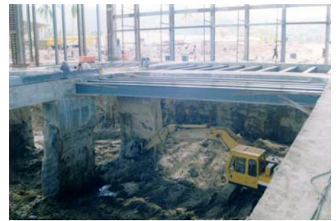
Basement excavation in progress, using Top-Down Method.
