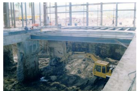
Basement excavation in progress, using Top-Down Method.
