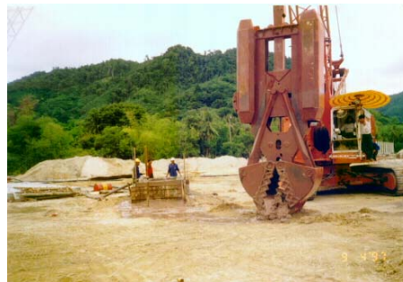
Excavation for a barrette.
