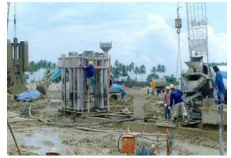
Casting a diaphragm wall panel.
