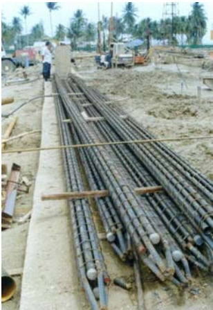
Anchor piles installation in progress (by other).
