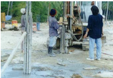
Anchor piles installation in progress (by other).
