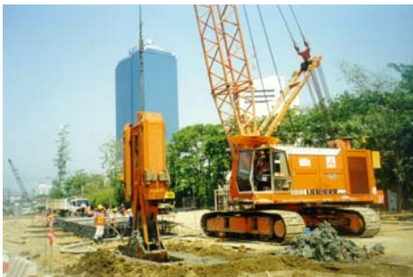
Panel excavation with grab.
