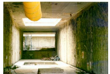
TBM retrieval shaft and cut & cover tunnel.
