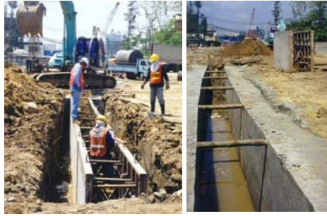
Guide wall construction.
