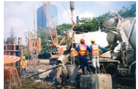
Concrete pouring using double tremie sets for a 4.5m long panel.
