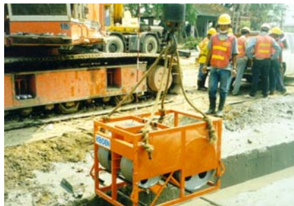
Koden drilling monitoring equipment in position for checking trench verticality.
