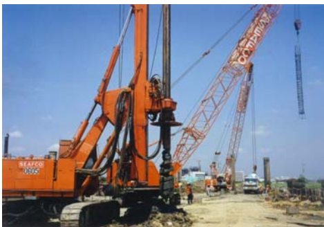
Bored piling in progress.
