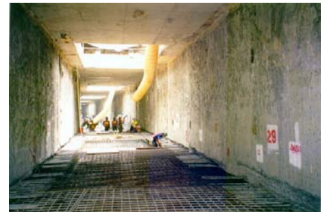
Cut and cover tunnel.
