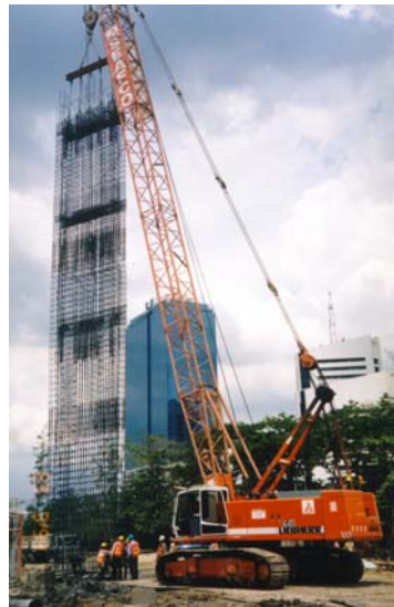
Lowering a 25.5m long reinforcement cage into the excavated trench.
