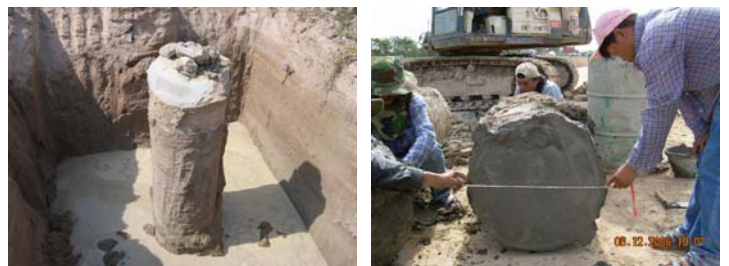
Deep soil mixing (soil-cement column works) in progress.
