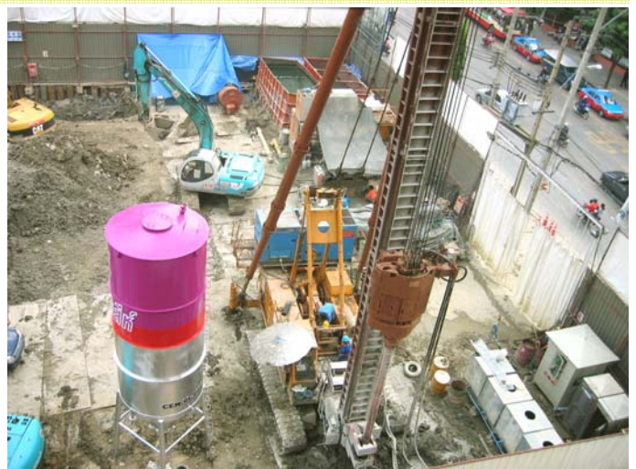
Improvement of soft clay with soil-cement column construction.
