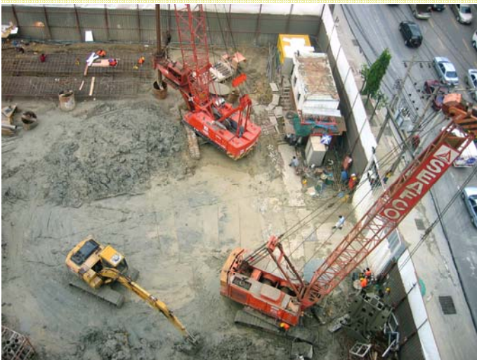
Diaphragm wall and bored pile construction in progress.
