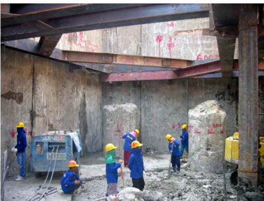
Excavation reached to the final depth of about -11.0m.
