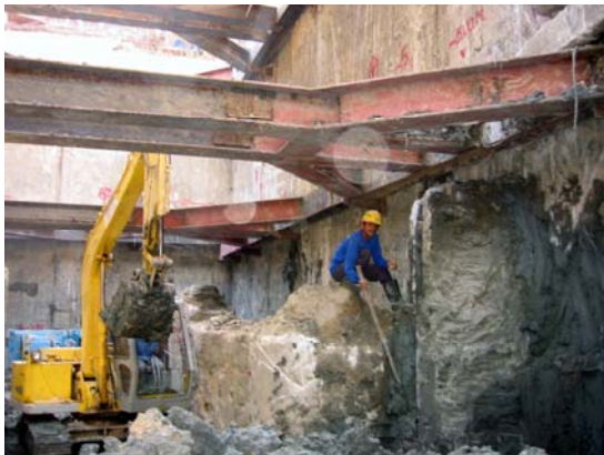
Exposed soil-cement columns below 2nd bracing layer.
