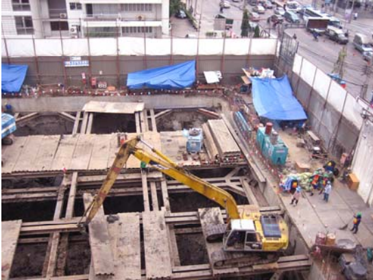
Excavation work with temporary bracing in progress.
