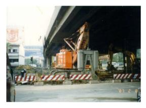
Diaphragm wall panel excavation with modified grab crane under the existing expressway.
