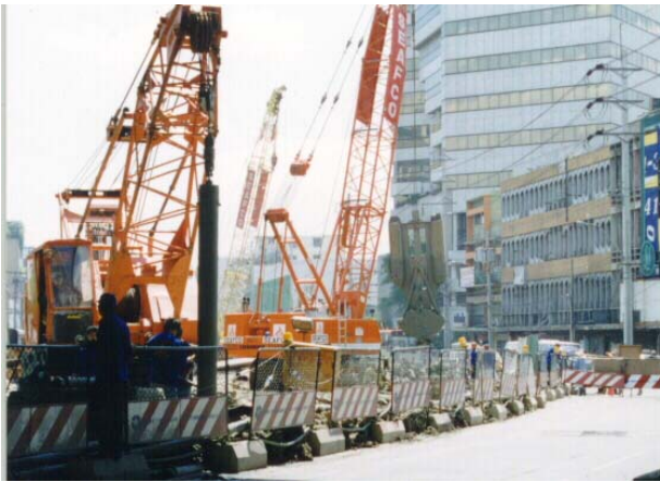
Diaphragm wall panel excavation in the middle of traffics.
