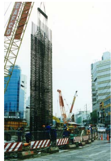
Lowering a rebar cage section.
