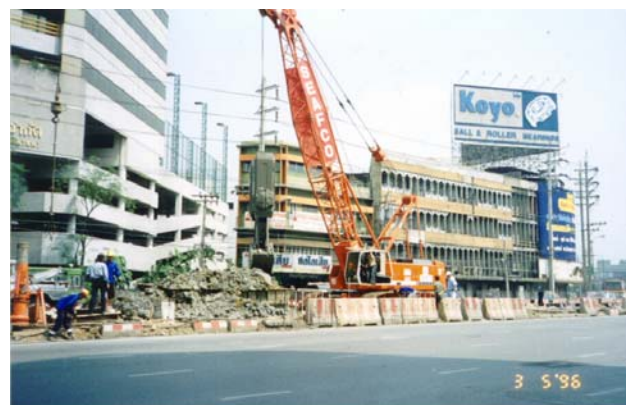
Diaphragm wall panel excavation in progress.
