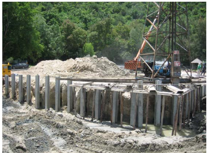
Installation of concrete facing walls for boat berth and ramp by other — soil retained by soil-cement columns.
