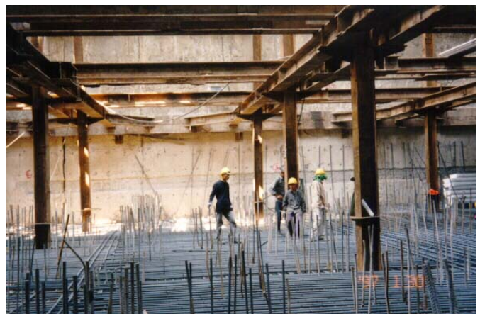
Base slab (mat foundation) at 15.0m below the ground.
