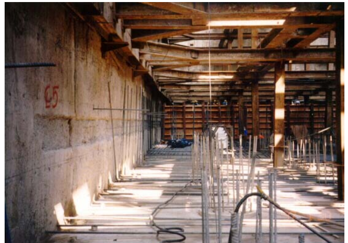
24m long reinforcement cage installation.
