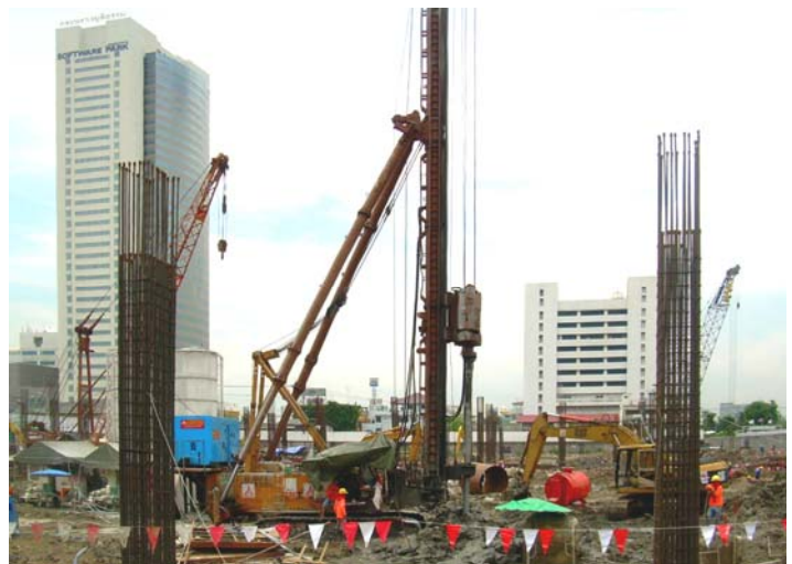
Deep soil mixing (soil-cement column works) in progress.
