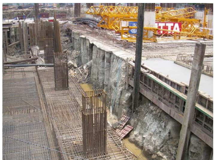
Soil retained by soil-cement columns for basement excavation and construction works.
