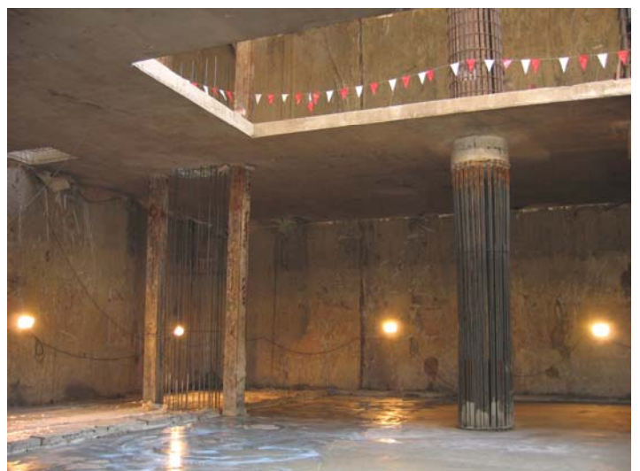
Exposed diaphragm wall faces, laterally supported by basement slabs.
