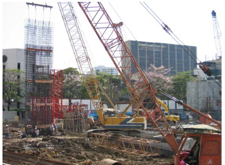
Diaphragm wall construction in progress.
