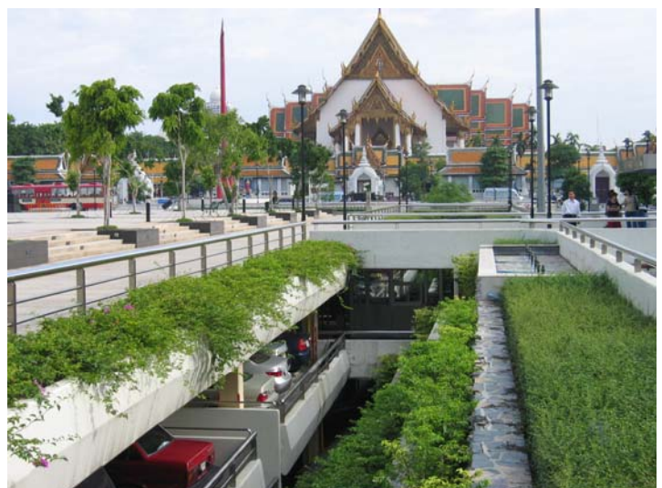
Completed Car Park.
