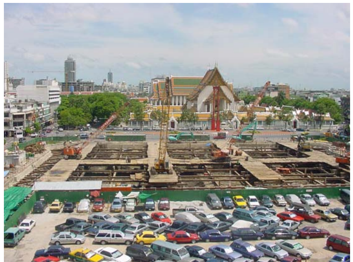
Excavation in progress.
