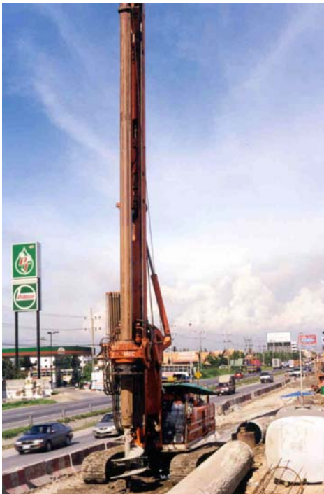
Bored piling along traffic median.
