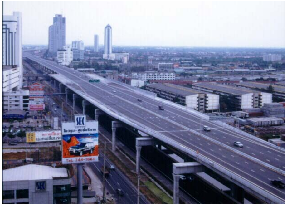
General view of expressway.
