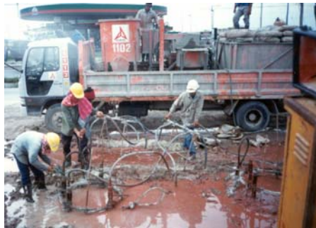
Pile base grouting in progress.
