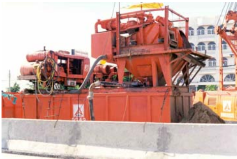
Bentonite plant for bored piling.
