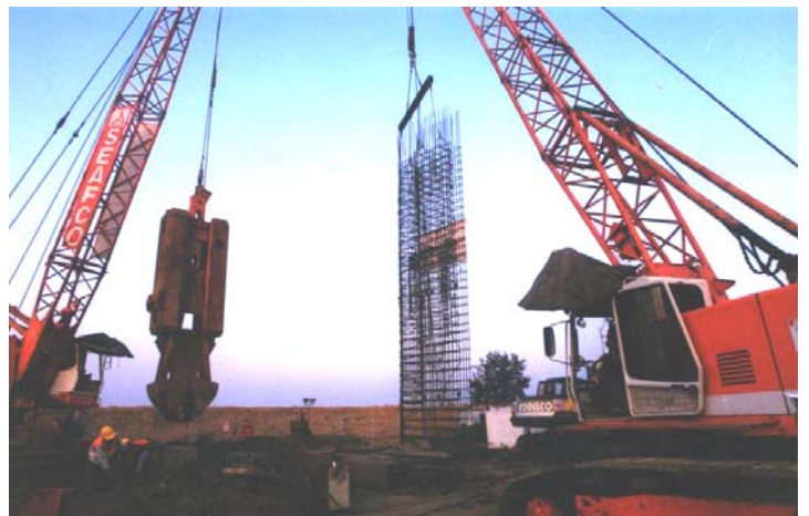
Diaphragm wall construction in progress.
