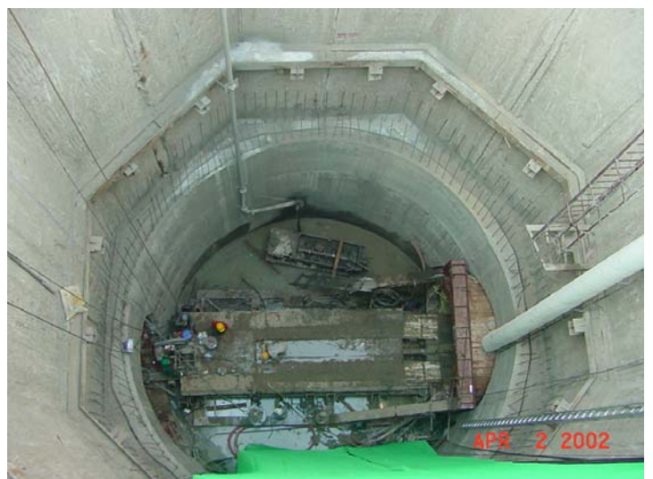
Circular shaft formed by diaphragm wall panels.
